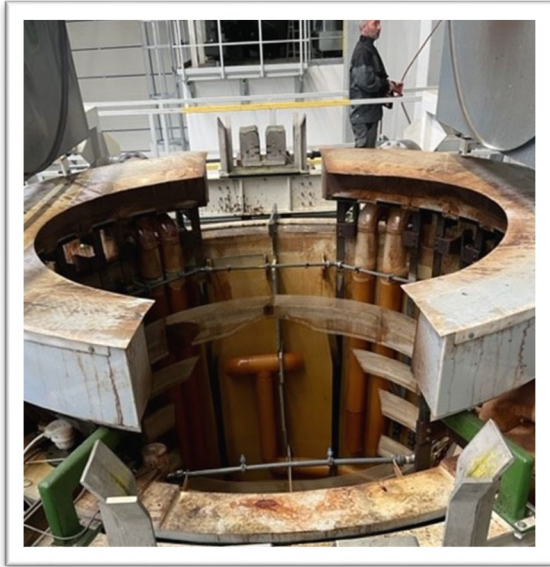
Closed 40,000 l reactor for chrome plating of valve balls for pipelines /20/
